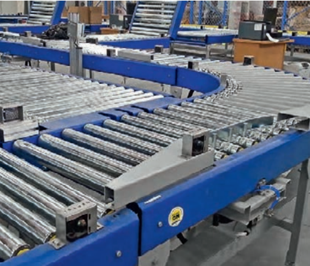
Neptek's intelligent conveying systems at ASCO, with Interroll rollers, drives and controls
