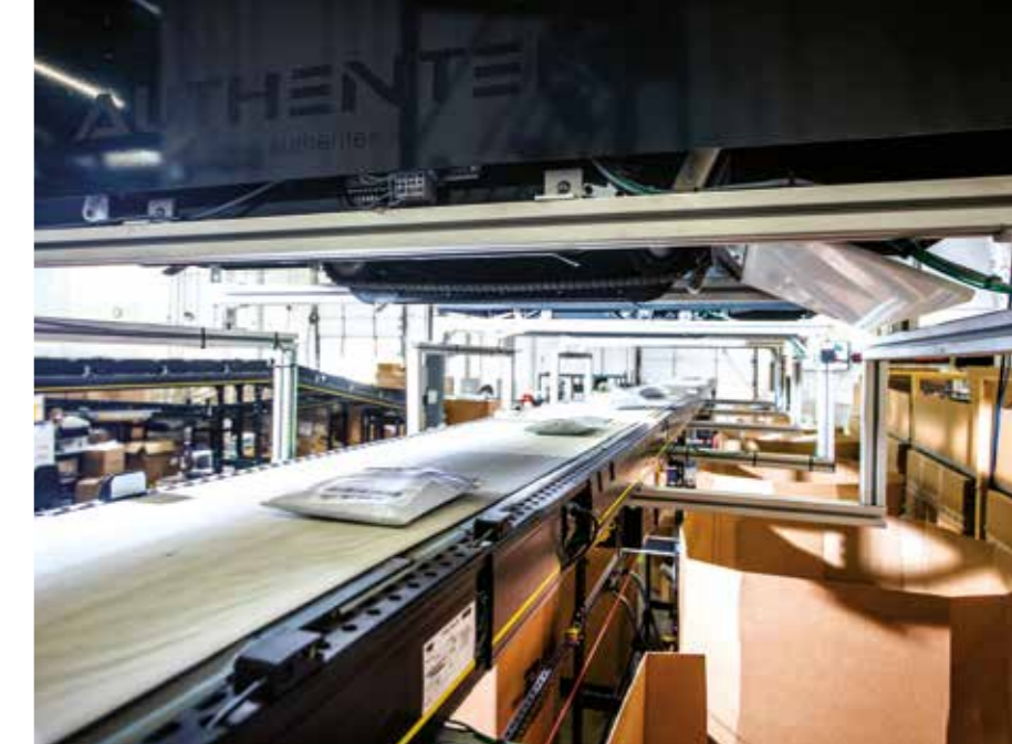
High throughput, large variety of goods: Automated material flow solution connecting the packaging and shipping areas at Shop LC.
